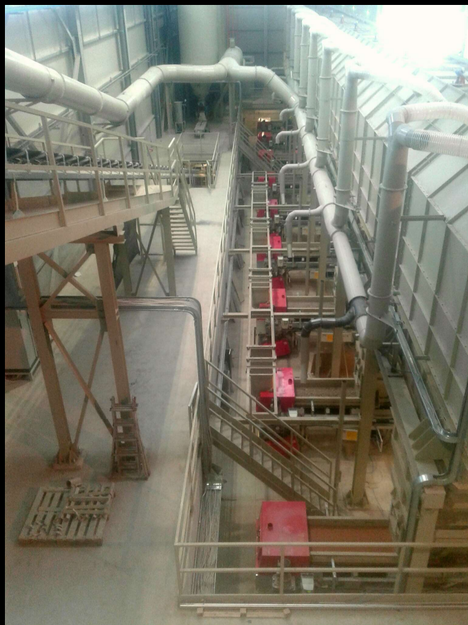
Line with raw material hoppers
