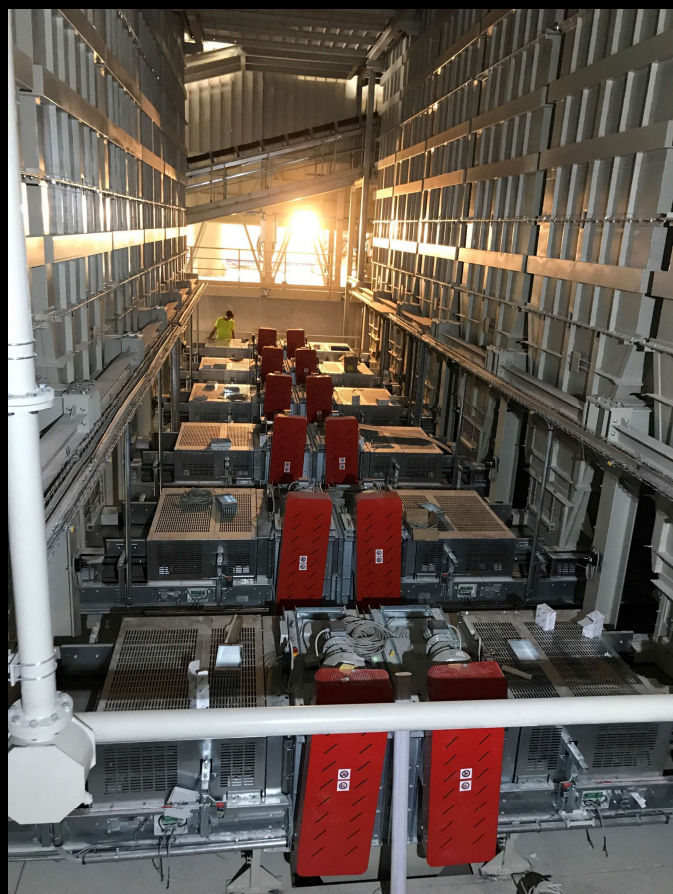
Line with raw material silos
